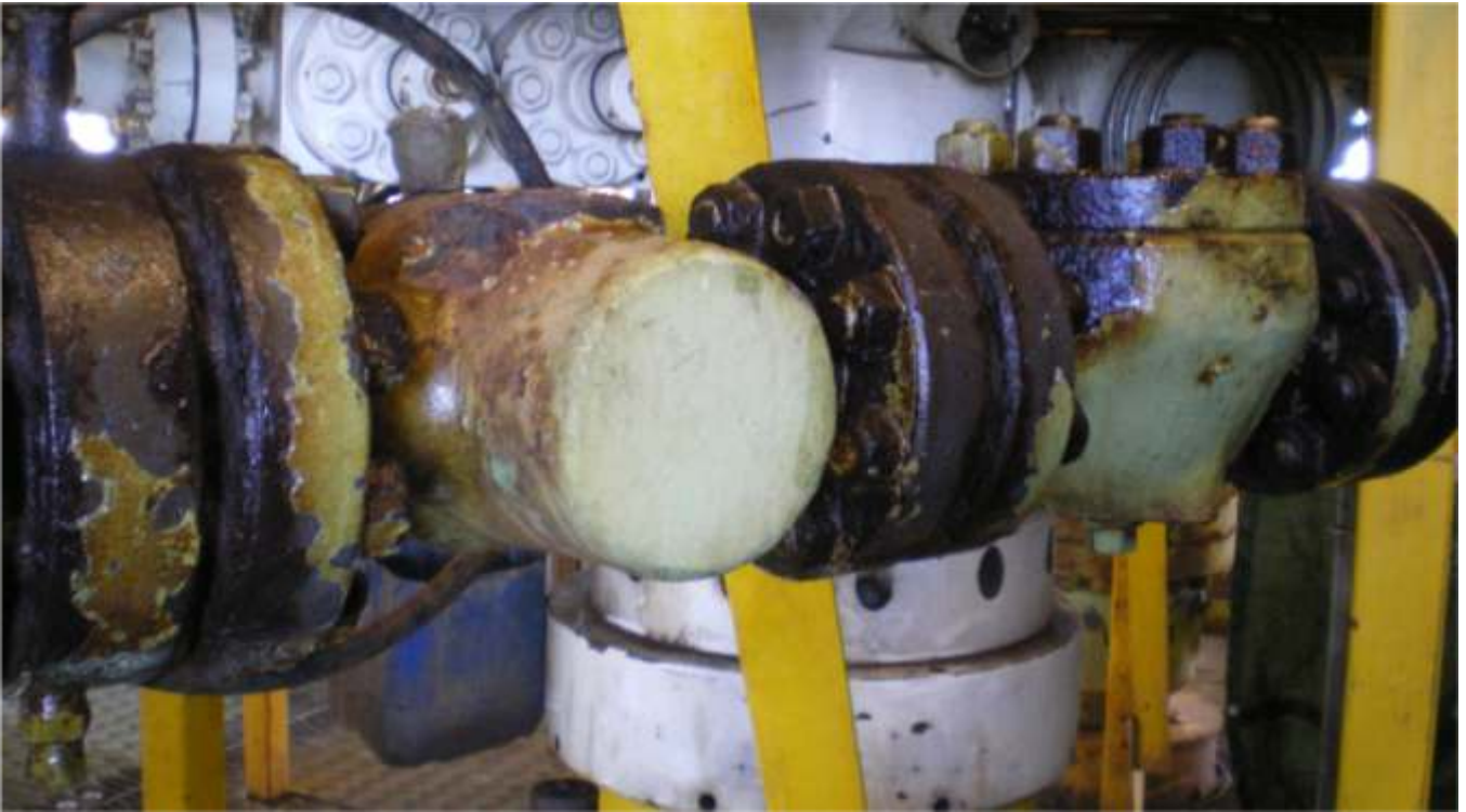
Above: a 'branch' of the christmas tree following removal of all unsound material.
