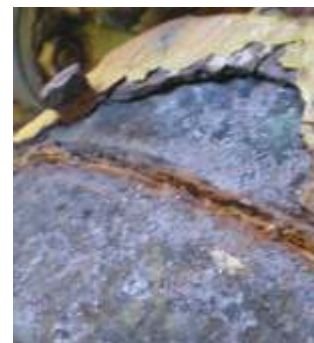
Below: preparation complete on small flange, ready for application of inhibitor.
