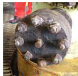
Below: preparation complete on small flange, ready for application of inhibitor.
