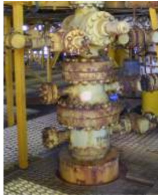
Left and below: platform viewed from the sea; well head showing heavy corrosion with closer details of corrosion effects on flanges and bolts.
