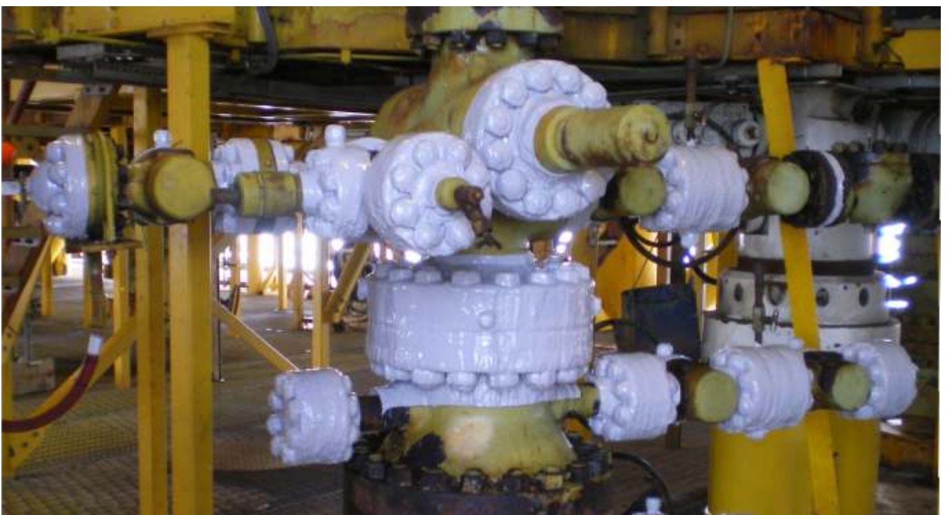
Below: completed sections graphically demonstrate the level of protection afforded by the Enviropeel encapsulation.
