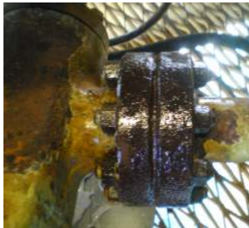
Above: a 'branch' of the christmas tree following removal of all unsound material.
