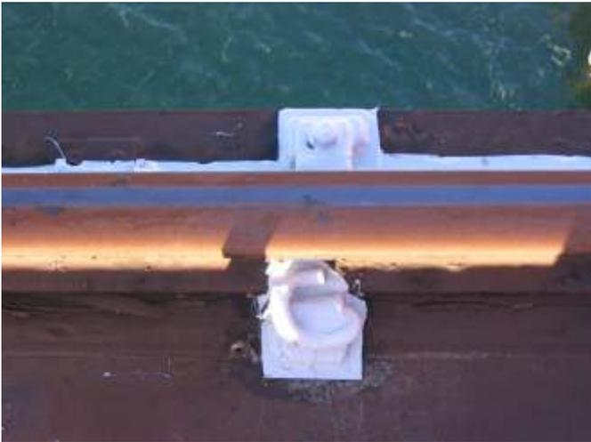
Top: A single cleat and pigtail prior to coating
