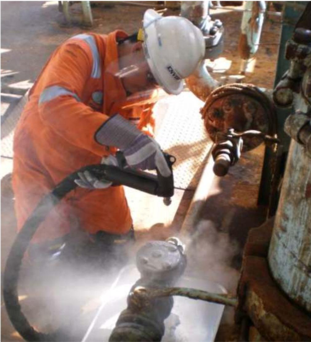
Surface preparation for the flanges and assembly was by air-powered needle gun and wire brush, removing all rust flakes to get the surface to a good application standard.
