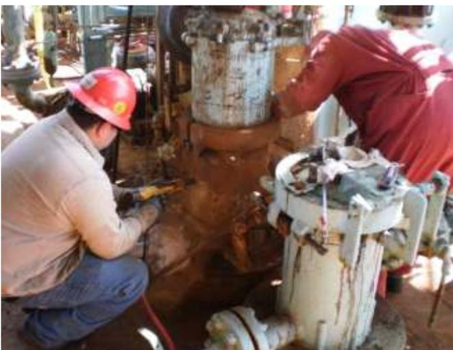
Before application the substrate is cleaned using needle guns and wire brushes.
