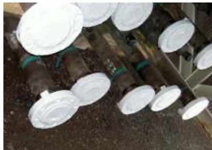
Secondly, built-in inhibiting oils that are constantly released on to the inner surfaces of the encapsulation provide constant corrosion protection.
