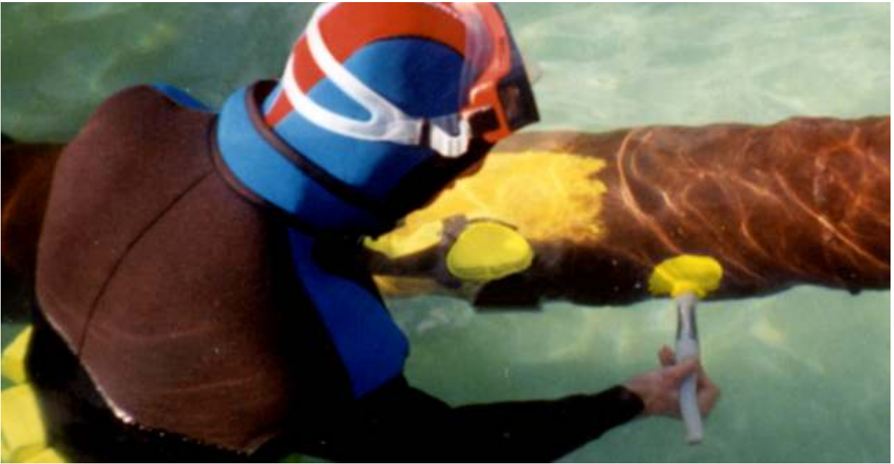
Above: Brush application in the splash zone
