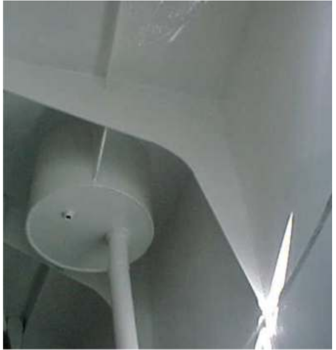
Above: Inside the coffer dams after coating Above left: Buoy bottom after hydro blasting Left: Stripe coating cofferdam with 28.15
