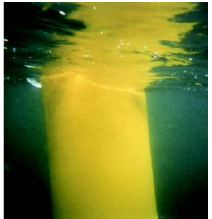
Below: Underwater, the leg can be seen to be fully coated and protected.
