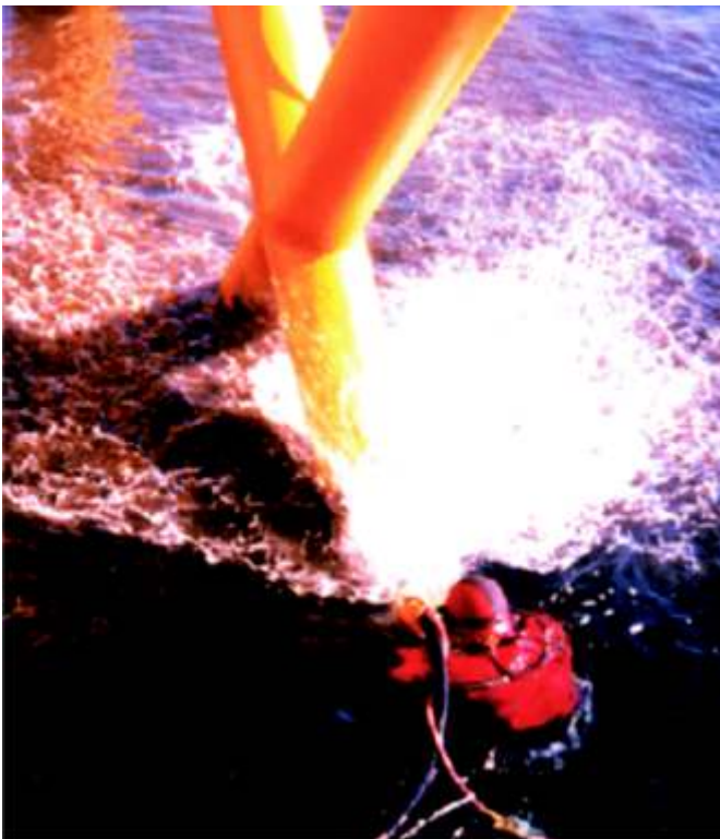
Top left: A diver prepares the surface for coating using grit-blasting equipment.
