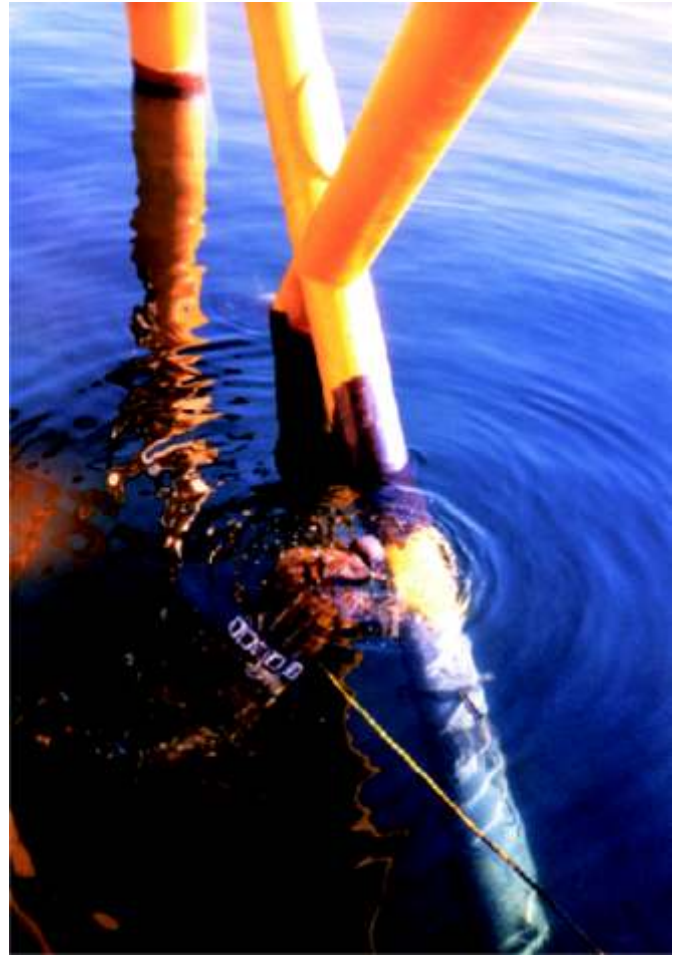
Top left: A diver prepares the surface for coating using grit-blasting equipment.
