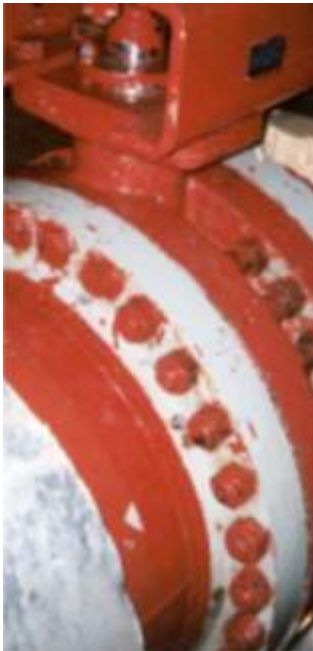
Above: Flange surface after preparation.
