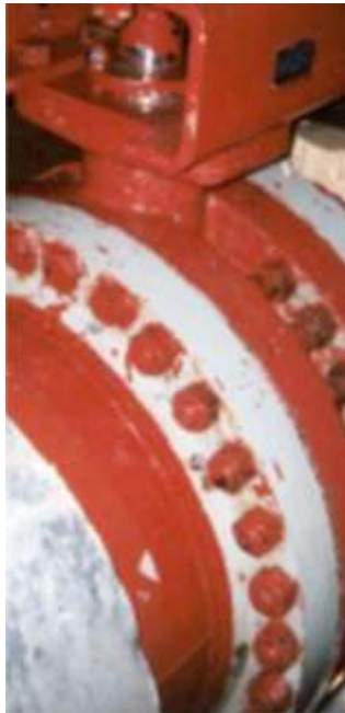
Above: Flange surface after preparation.
