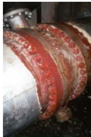
Above: 32" flange after removal of insulation.
