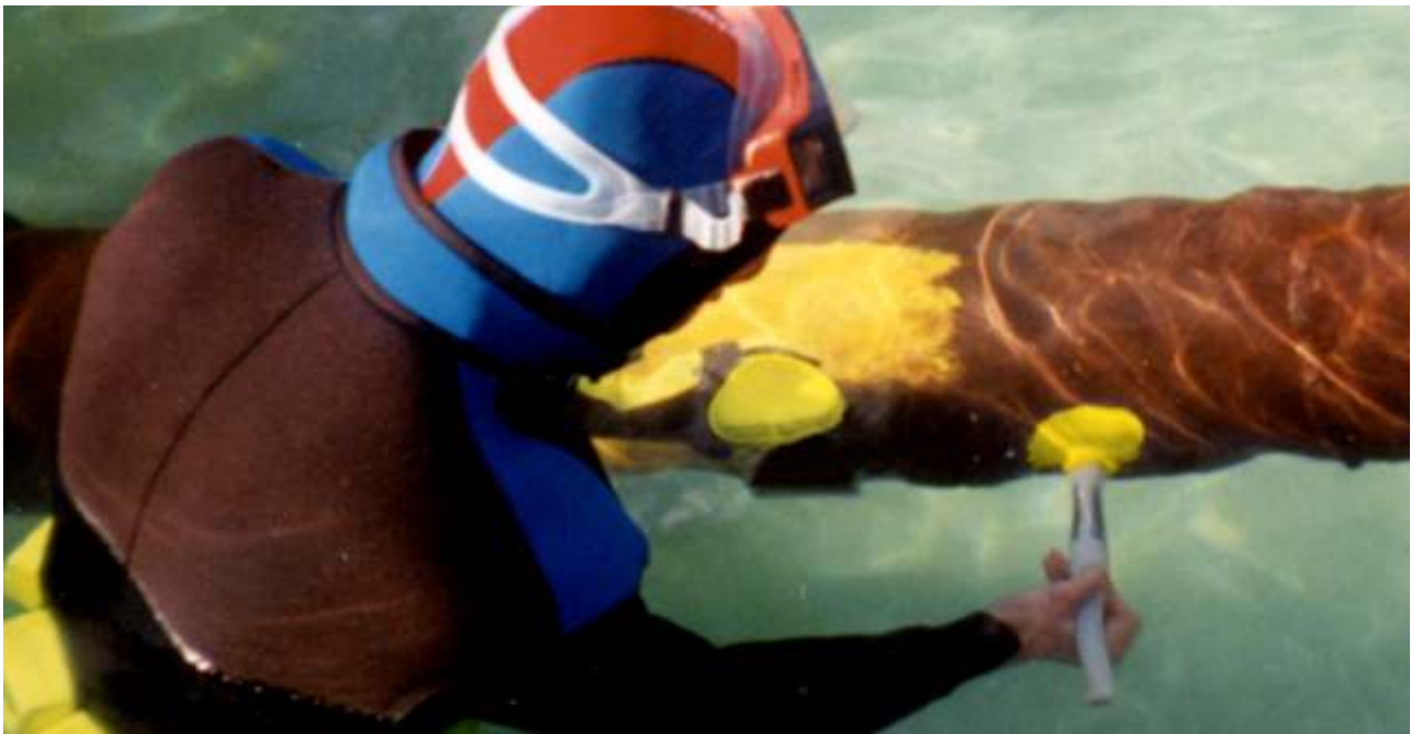
Above: Brush application in the splash zone
