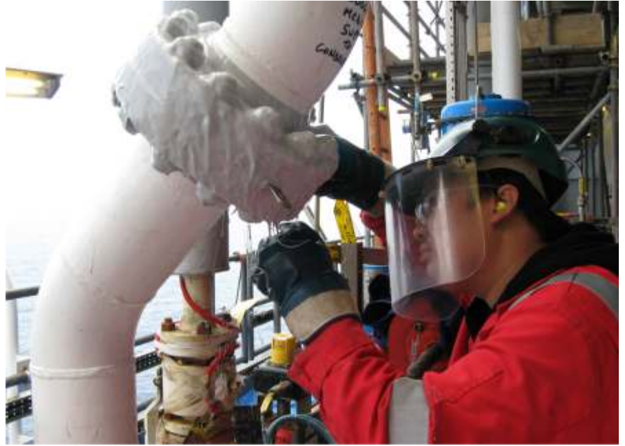
Application builds coats in succession, working from underneath, around the sides and finally above with two coats to provide maximum protection. The underside is the most difficult area to finish aesthetically but trimming between and after each coat ensures full protection. All trimmings and drips/spills are collected and recycled.
