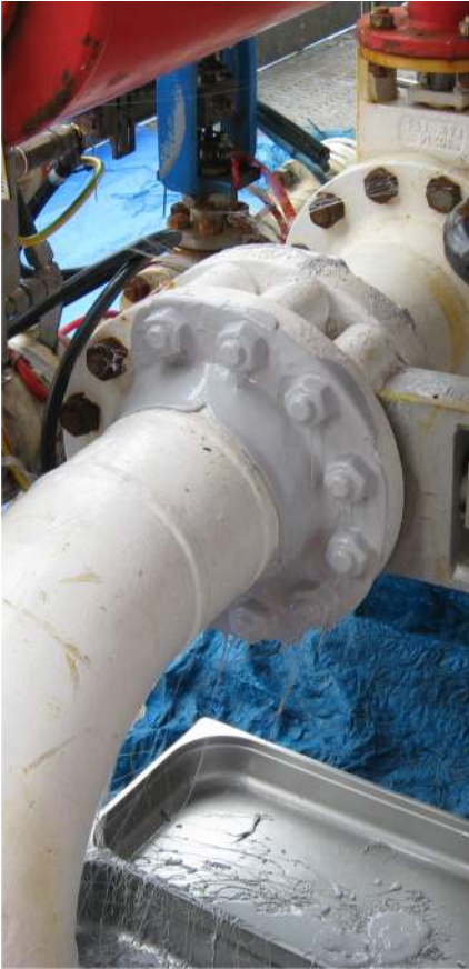
Application builds coats in succession, working from underneath, around the sides and finally above with two coats to provide maximum protection. The underside is the most difficult area to finish aesthetically but trimming between and after each coat ensures full protection. All trimmings and drips/spills are collected and recycled.
