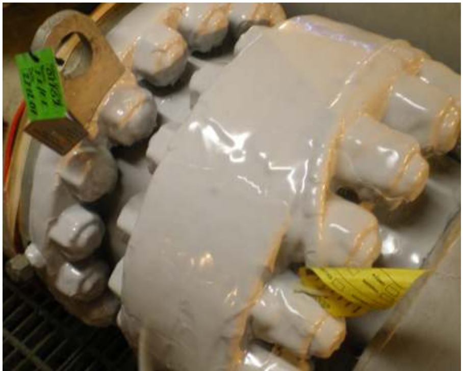
Application builds coats in succession, working from underneath, around the sides and finally above with two coats to provide maximum protection. The underside is the most difficult area to finish aesthetically but trimming between and after each coat ensures full protection. All trimmings and drips/spills are collected and recycled.
