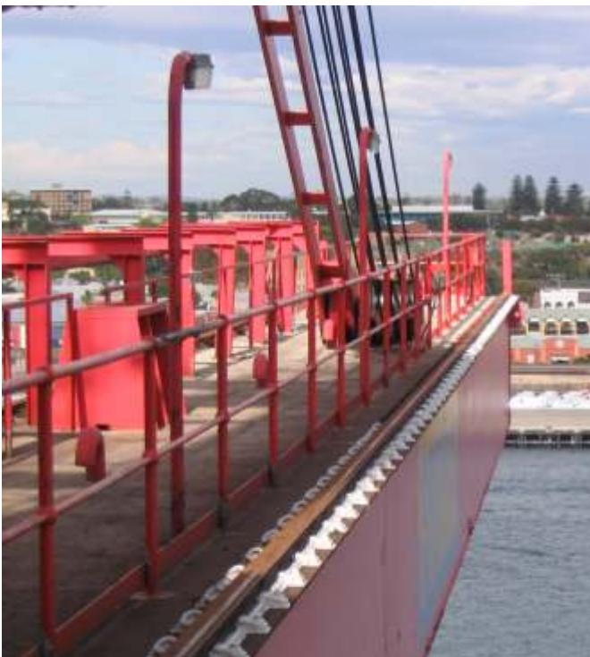
Right: A length of track on the jib showing coated cleats linked with Enviropeel to improve security Below Right: Views of Enviropeel coated cleats
