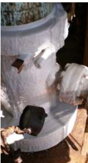
Right and below: the corrosion-inhibiting layer of Enviropeel provides a perfect way of preventing any further damage to the ageing platform infrastructure.
