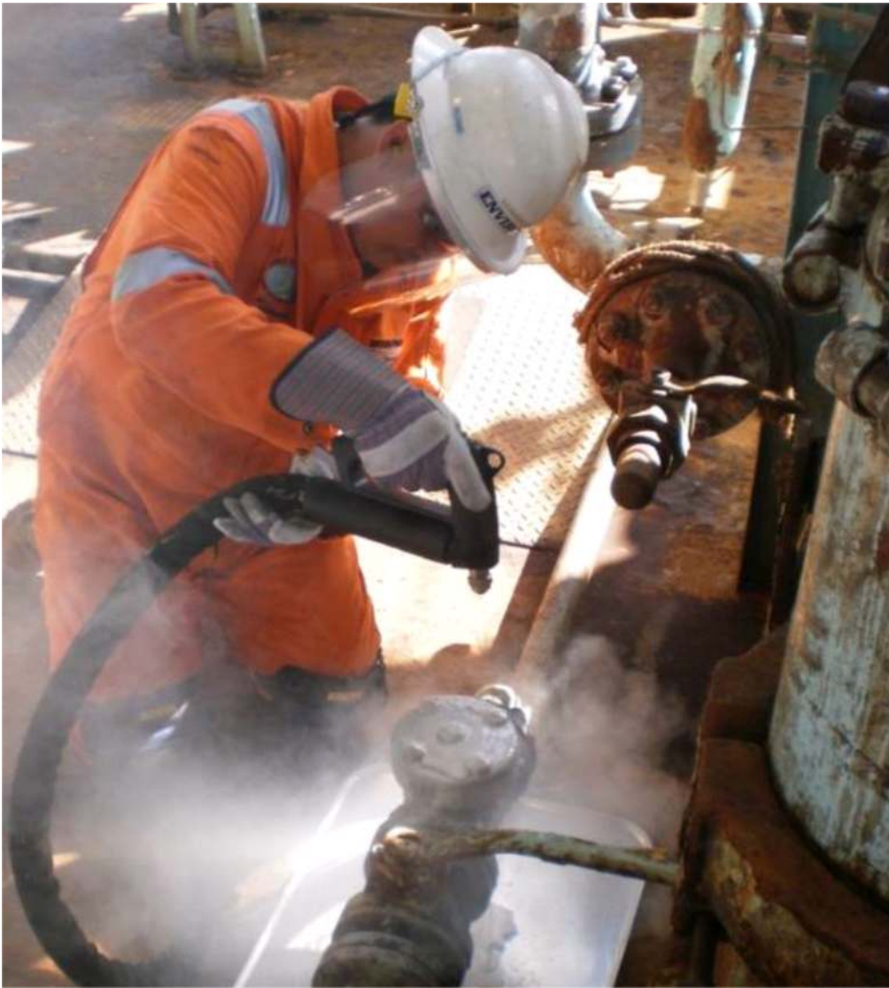
Top: Enviropeel personnel applying the system to prepared flange joints
