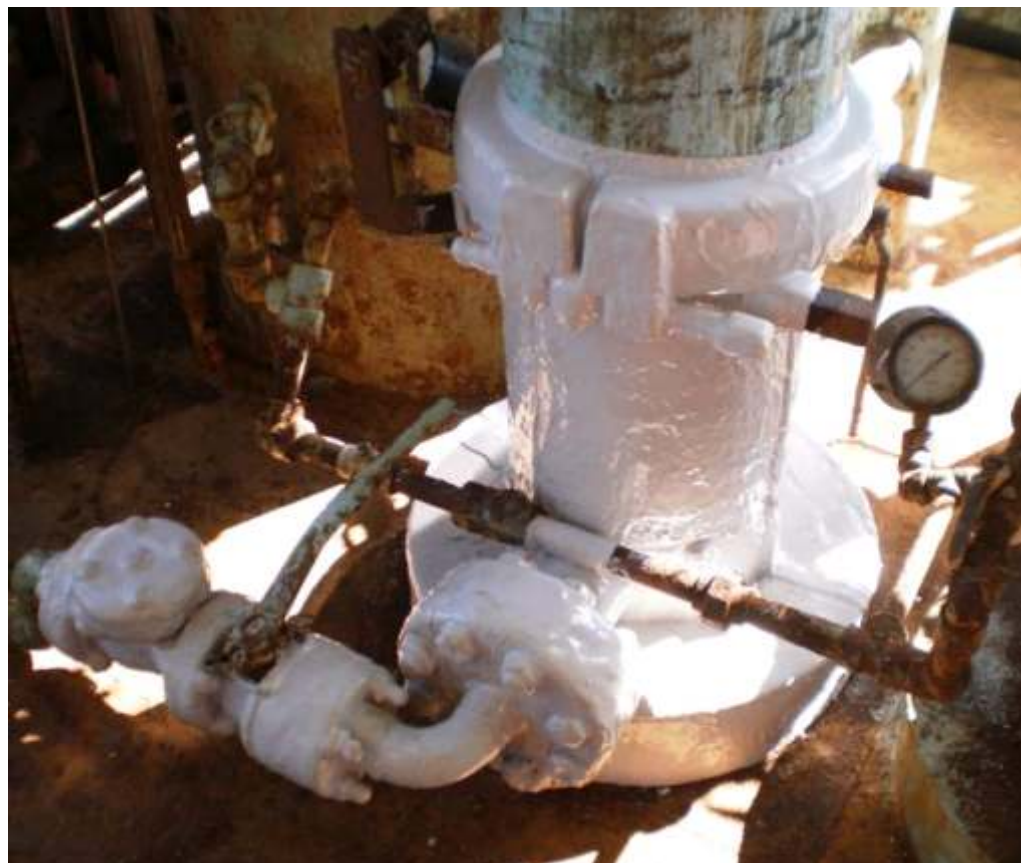
Right and below: the corrosion-inhibiting layer of Enviropeel provides a perfect way of preventing any further damage to the ageing platform infrastructure.
