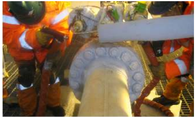
Left: A large a complex application on board an LPG tanker Above: Applying from both sides of larger flanges speeds up the operation and helps provide higher coating quality
