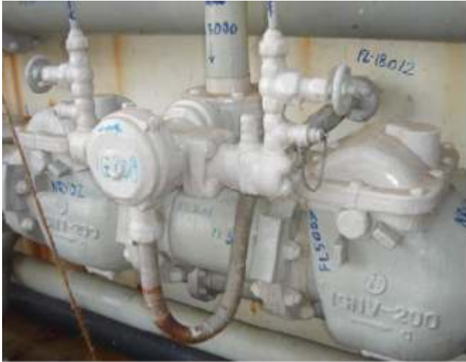
Left: A large a complex application on board an LPG tanker Above: Applying from both sides of larger flanges speeds up the operation and helps provide higher coating quality
