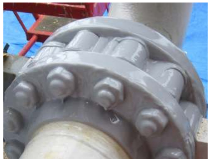
Below: a typical flange, perfectly encapsulated with Enviropeel to preserve its integrity.
